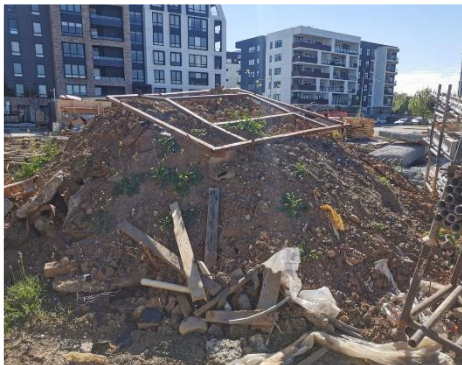
5. Overview of Stockpile SP1 located in the northern portion of the Site.
