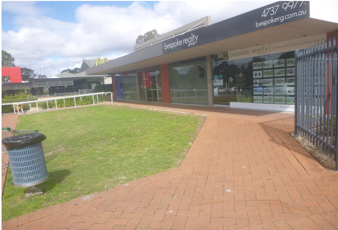
Photo 1: Commerical building at south of site
