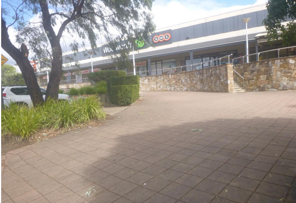
Photo 5: Retaining walls at site
