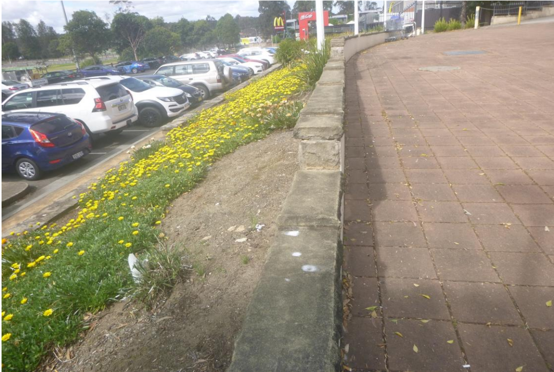
Photo 3: Batter slope near western site boundary
