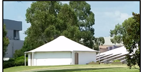
Photograph 6 – Detached toilet block
