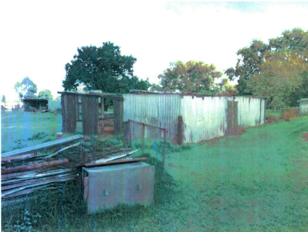
Figure 2 - The shed in the context of the service yard area aligned with a yard fence showing the front clad with corrugated sheeting and rear portion built of timber slabs.
