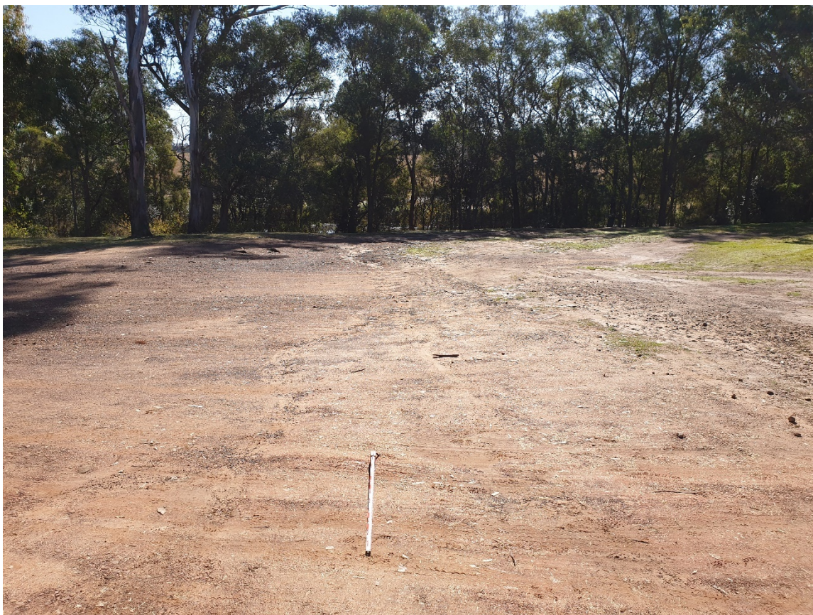
Figure 5.7 North facing view showing widespread sheet erosion on hill slope (1m scale).
