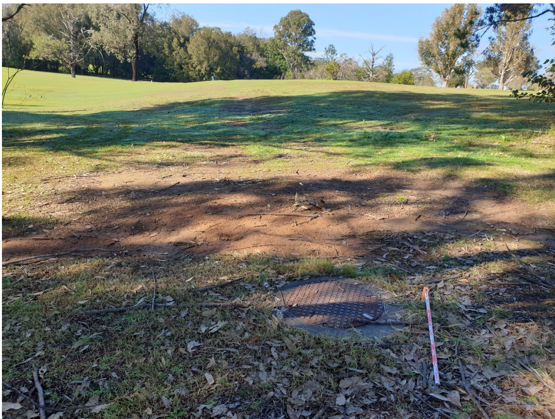
Figure 5.4 North-east facing view showing manhole cover (1m scale).
