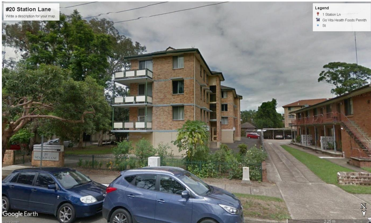
Figure 7 Street View showing four storey development at #20 Station Lane to the north of the subject site (image courtesy of Google Earth Pro)
