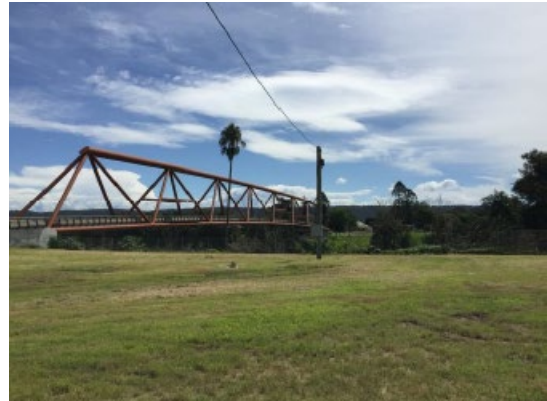
Figure 6 View east from Lot 21 towards pedestrian bridge
