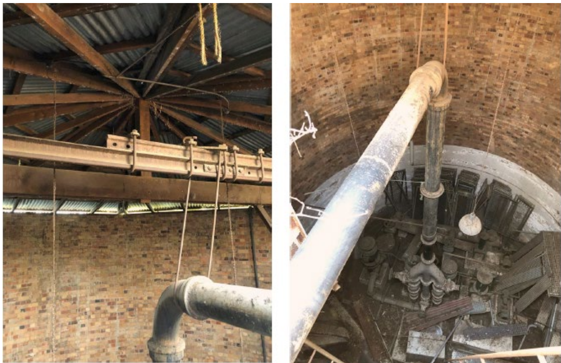
Figure 12 Interior of the remnant Pump House
