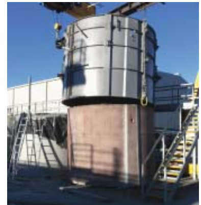
A CABS tank being de-moulded
