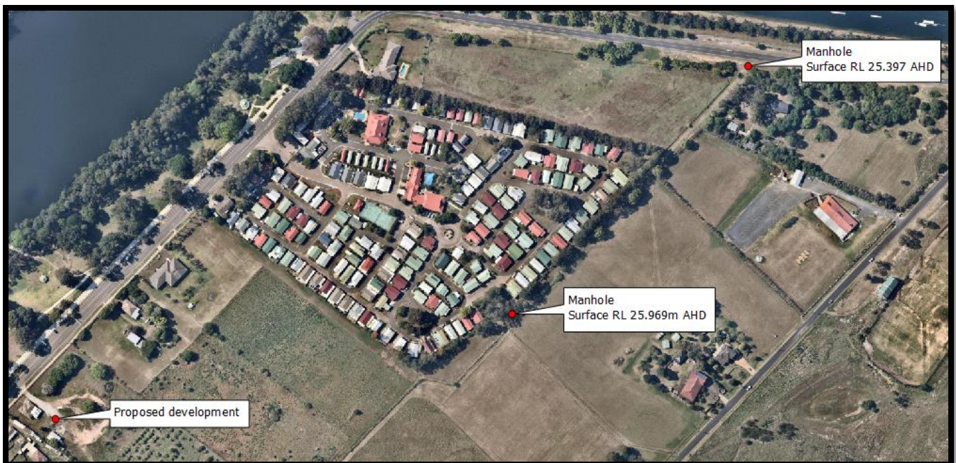
Figure 3 Closest manholes to the development
