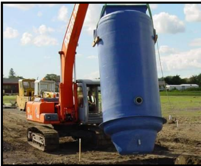
Figure 10 Package pumping station wet well to be buried on site
