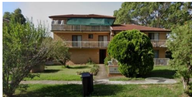
Figure 11 - South view looking into property at 8 Railway Street - i.e. the east adjoining site (google street view image Jan 2019)
