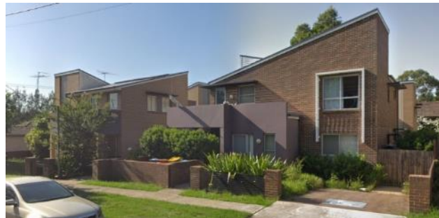
Figure 12 - South view looking into property at 6-7 Railway Street - i.e. the further east adjoining site (google street view image Jan 2019)
