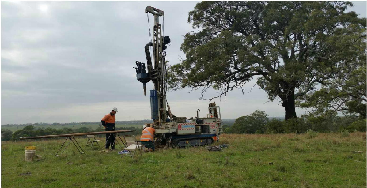
Photo 13: BH14 Drill rig set up looking east
