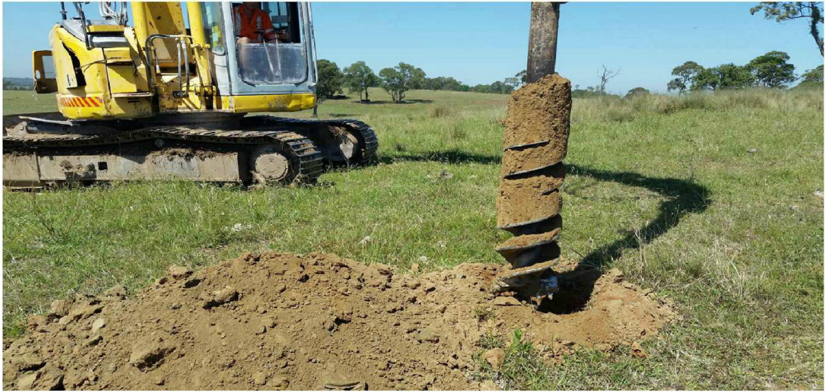
Photo 1: 14 tonne excavator with pendulum auger at BH09 south
