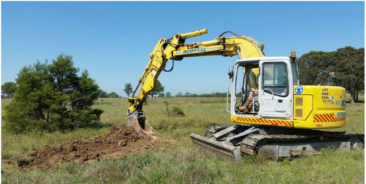
Photo 3: 14 tonne excavator at TP13 looking south
