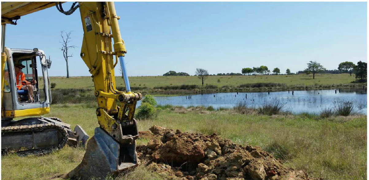
Photo 4: 14 tonne excavator at TP14 looking north east
