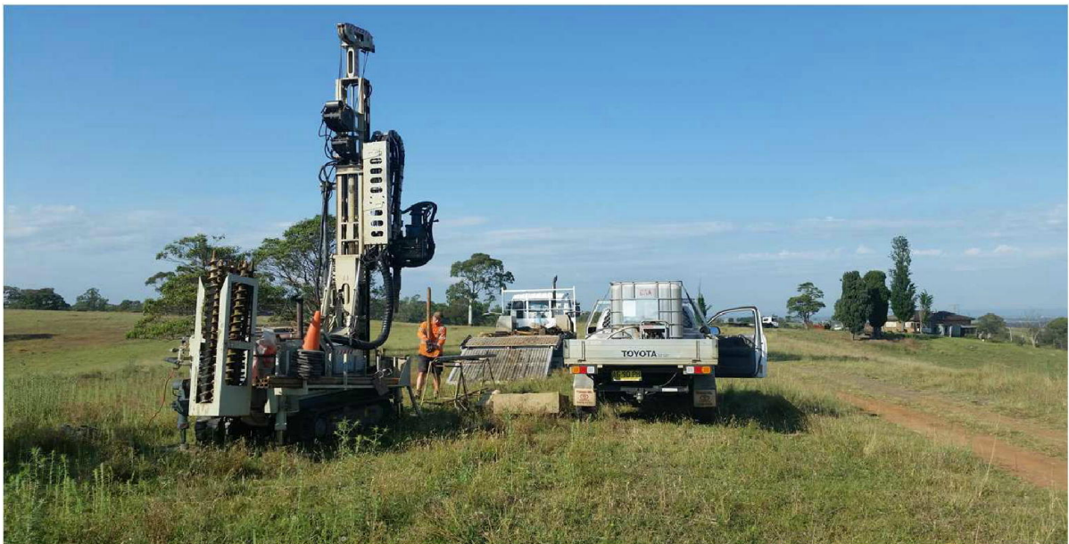
Photo 14: BH15 Drill rig set up looking south
