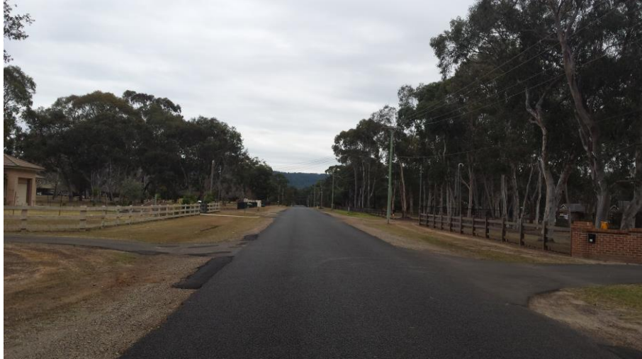
Looking west along Jolly Street
