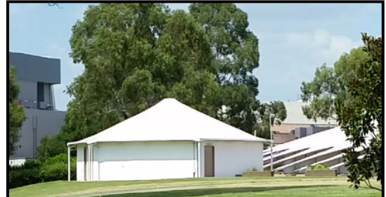
Photograph 6 – Detached toilet block
