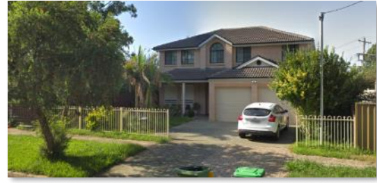
Figure 12. Development at 14 Railway Street, Werrington (Source: Google Maps Street View).
