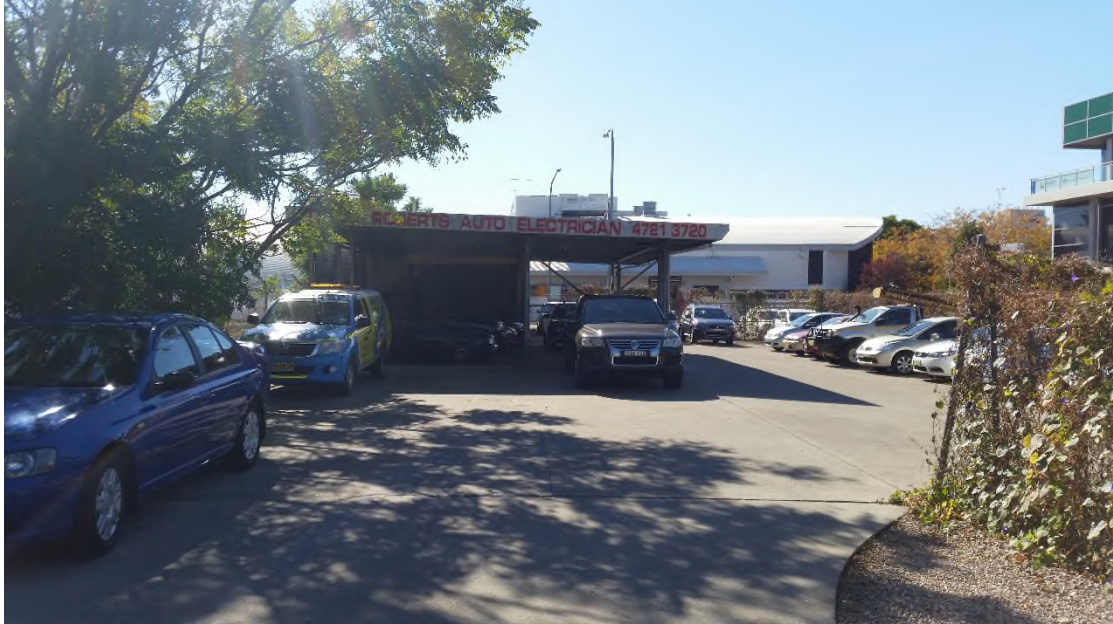
Photograph A3.1: Disused structure and vehicle parking on the subject site
