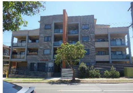
Figure 12 - View looking east towards 207 Derby Street, a recent four-storey residential development.
