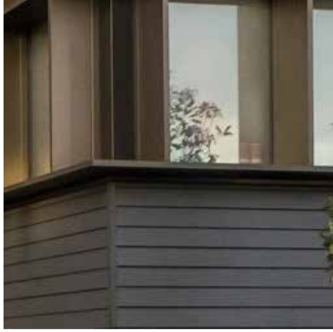
FC - 01 PANELISED WALL CLADDING WITH HORIZONTAL GROOVE
