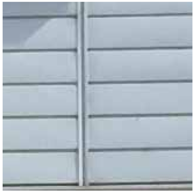
INSULATED PANEL WITH EXPRESSED HORIZONTAL TEXTURE
