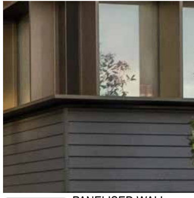
FC - 01 PANELISED WALL CLADDING WITH HORIZONTAL GROOVE
