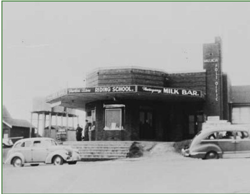
Figure 3.9 Photo of the new Wallacia post office in 1950 (NAA C4076, HN1071).
