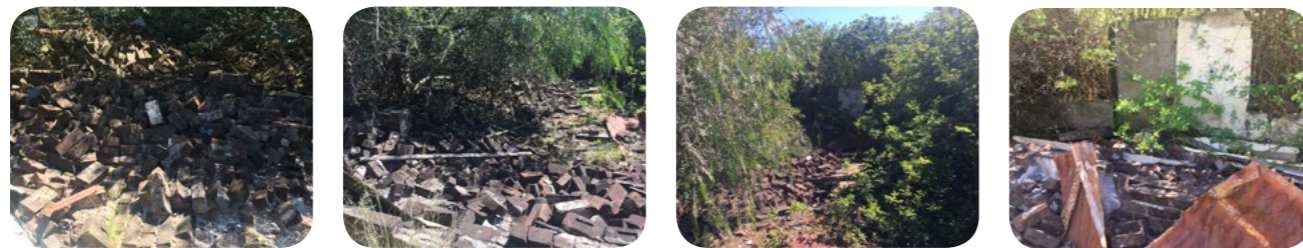
Reuse site material Recycled brick, approx. 500 usable bricks
