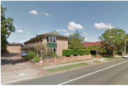
Derby Street townhouse development to the south
