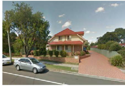
Derby Street townhouse development to the south
