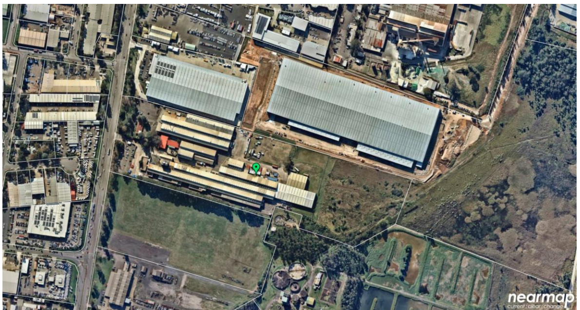
Figure 1.2. Aerial Imagery (Source: Nearmap 8 June 2020)
