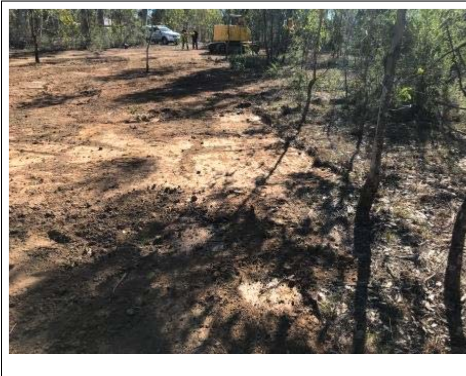
Image 7.1.2 View of stockpile SP02 removal footprint, facing north
