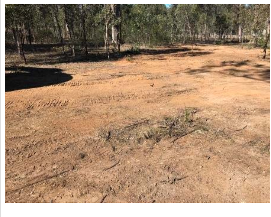
Image 7.1.2 View of stockpile SP03-SP11 removal footprint, facing south
