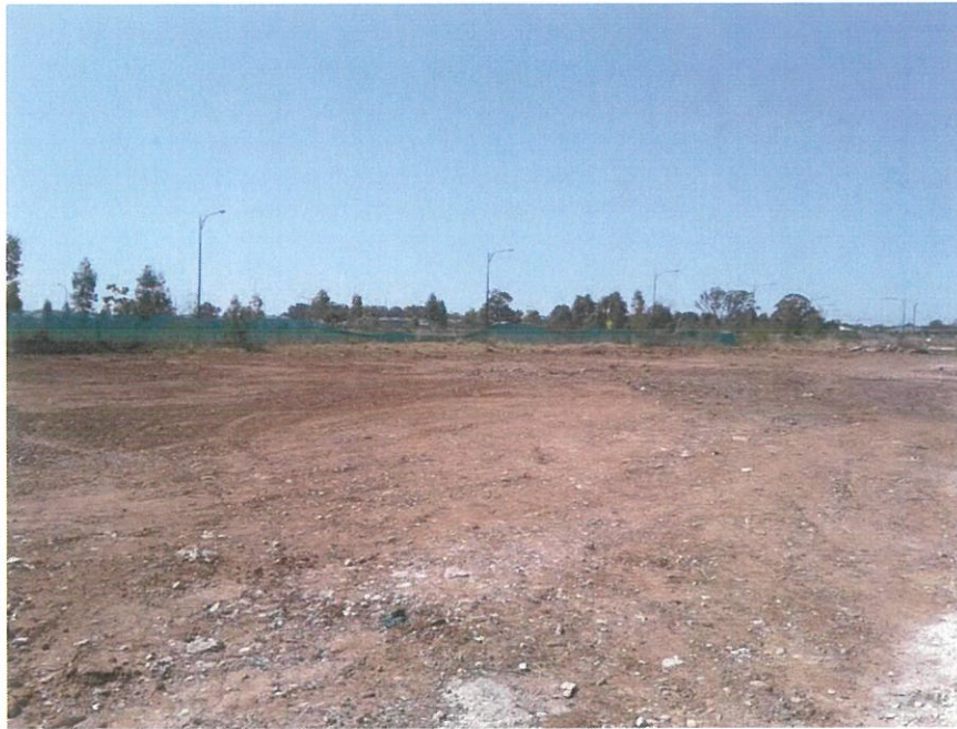
Photograph 7 - Filling in eastern portion of site
