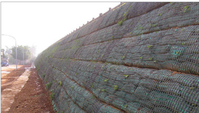
The use of ACEGrid® as a front wrapped reinforcement treatment and after completion showing the vegetated structure.
