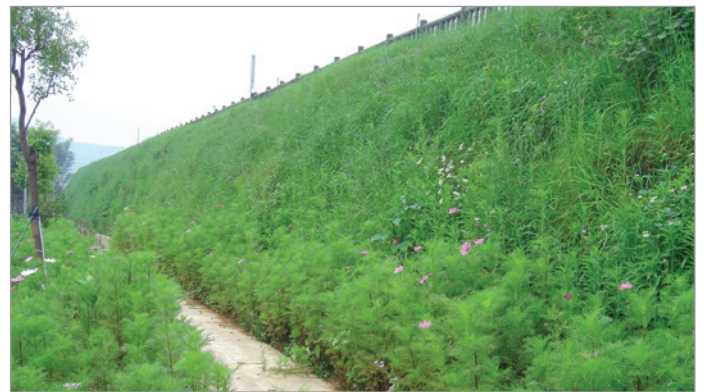
The use of ACEGrid® as a front wrapped reinforcement treatment and after completion showing the vegetated structure.
