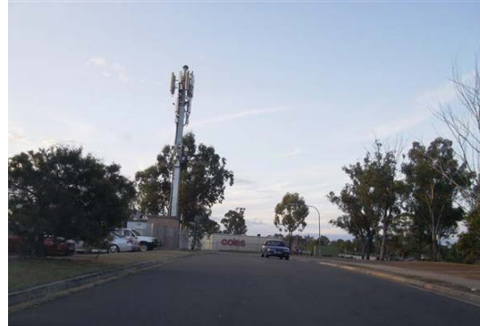
Figure 2.5: Boomerang Place (looking north along the eastern site boundary)
