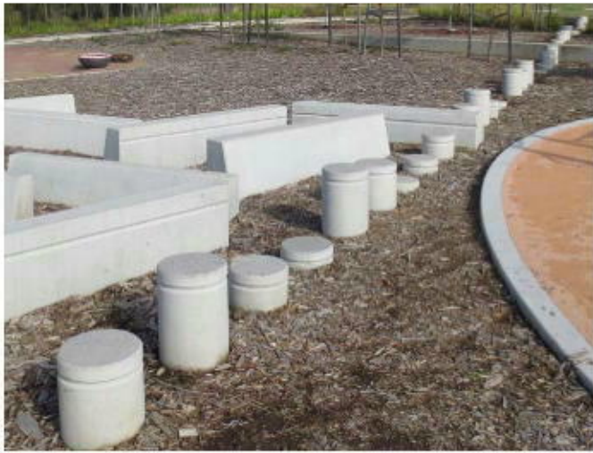
Concrete stepping stumps reduces the need for high levels of maintenance while still providing an interactive and challenging play element.
