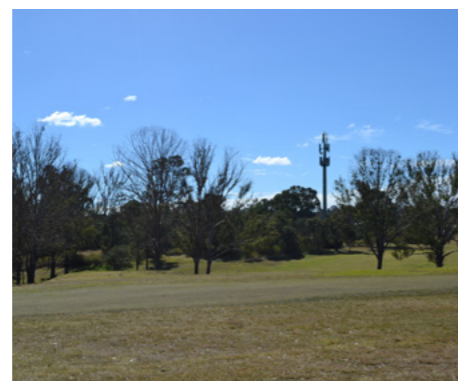
④ Telecom Tower
