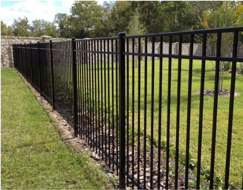
Figure 9: Typical security fencing
