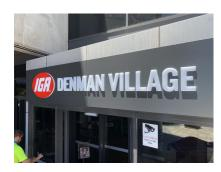
Light tray with LEDs then face installed
