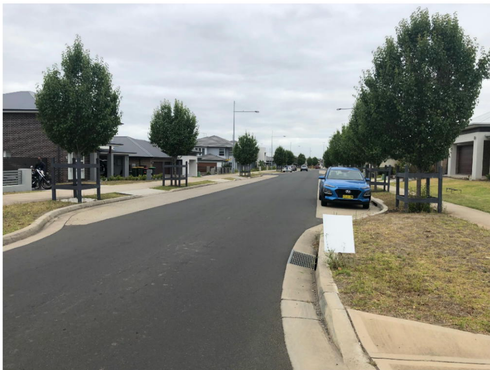
Figure 4a: Bradly Street facing East
