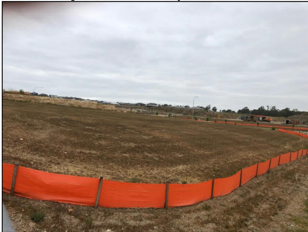
Figure 3: Photo of Development Site from Forestwood Drive
