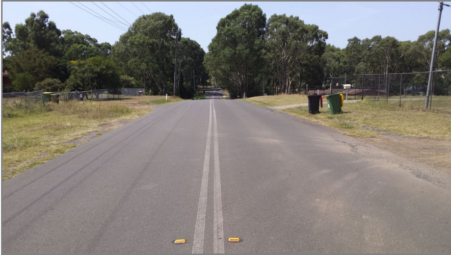
Photo 3: Mount Vernon Rd looking east
