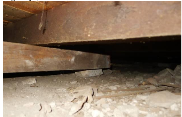
Figure 8: Typical view of floor substructure of Living Room Gallery.
