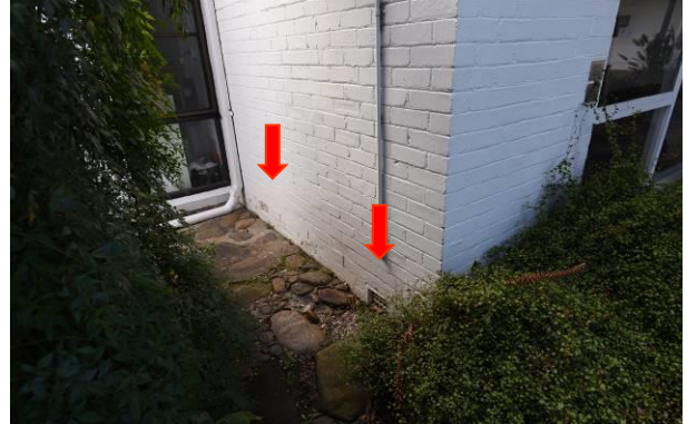
Figure 6: Existing ventilation grilles to northern wall of gallery (indicated).
