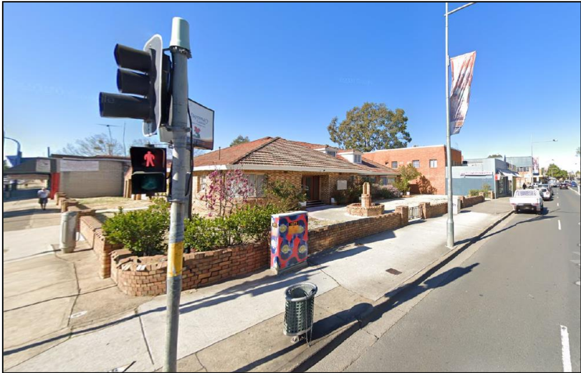
Image 1: View of the north-western corner of the site (former John Price & Son Funeral Home) looking from Station Street.
