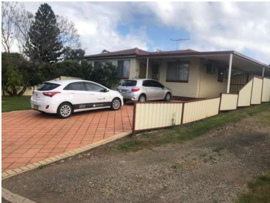
Figure 3b: Photograph of 32 Park Avenue
