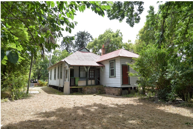
Figure 8 Cottage from south-west
