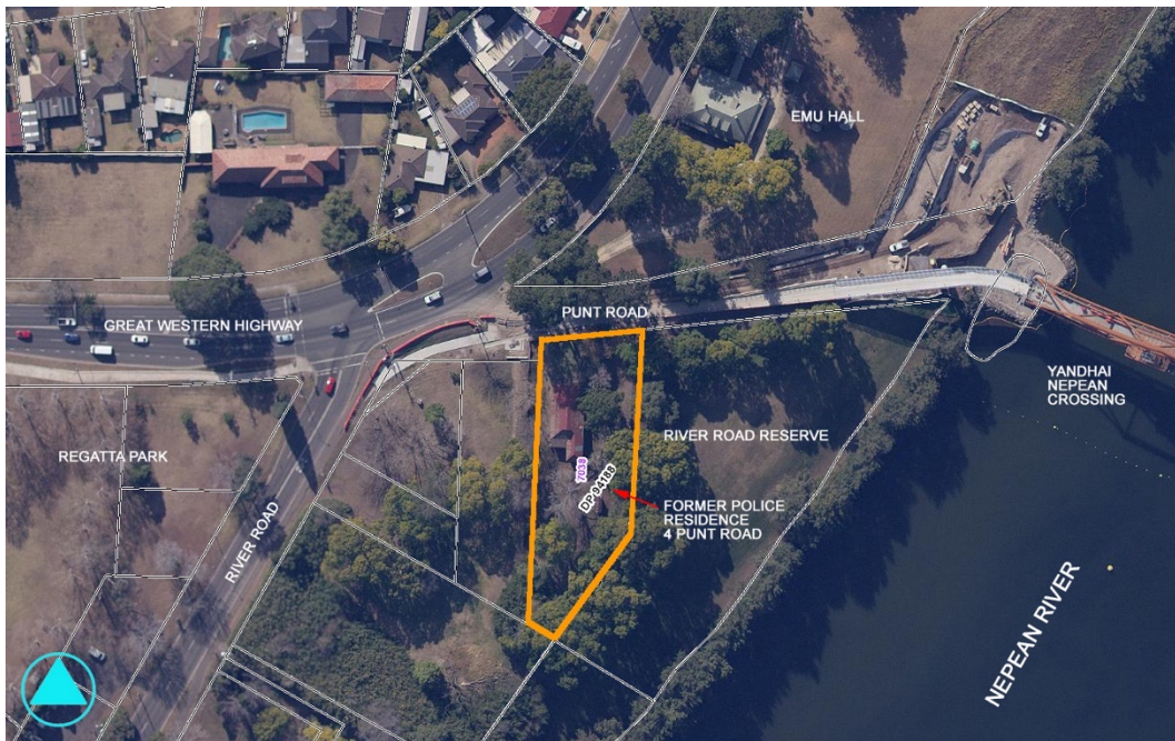
Figure 2 Aerial view of the subject property (outlined in orange) and the immediate locality. The real property definition of the place is Lot 7038, DP 94188. Source: SixMaps, 2020
