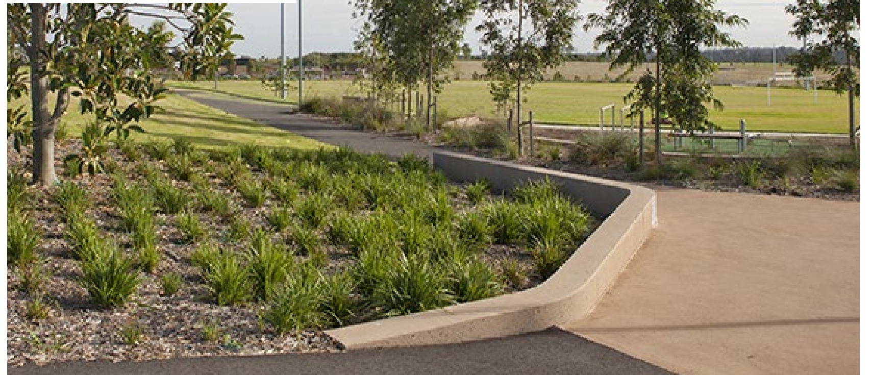
Insitu-Concrete Seating Walls
