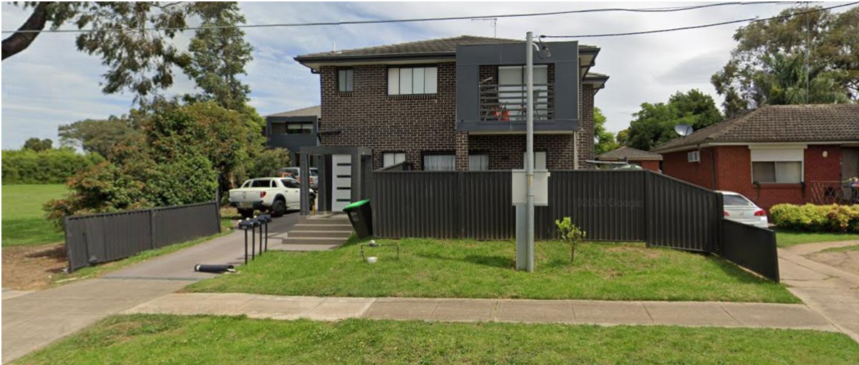
Image 5 – Multi dwelling housing at 66 Hobart Street
