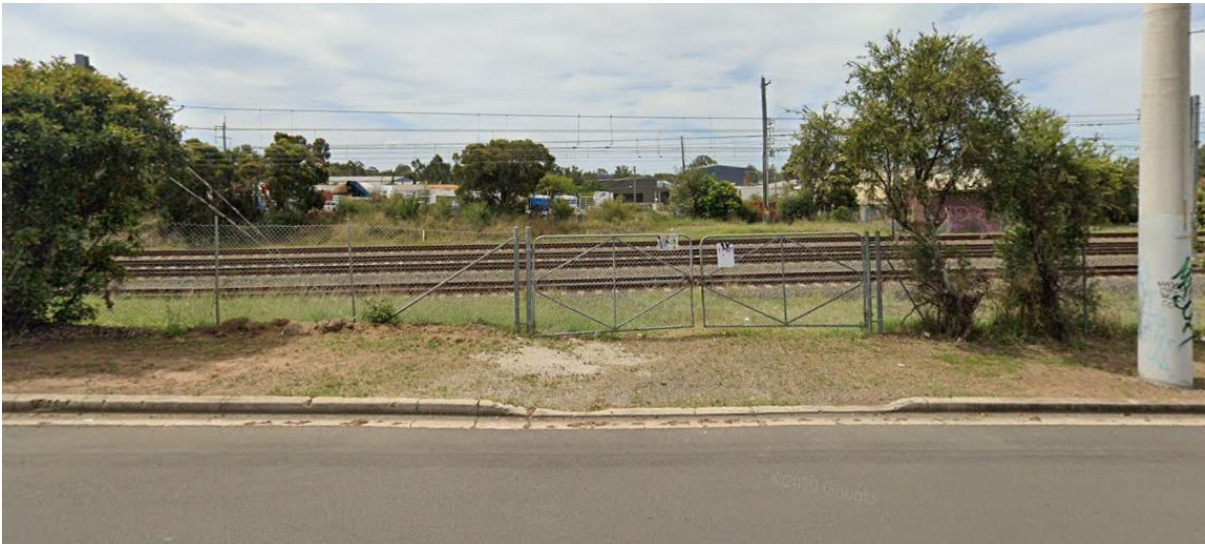
Image 6 – Sydney Trains asset across Hobart Street
