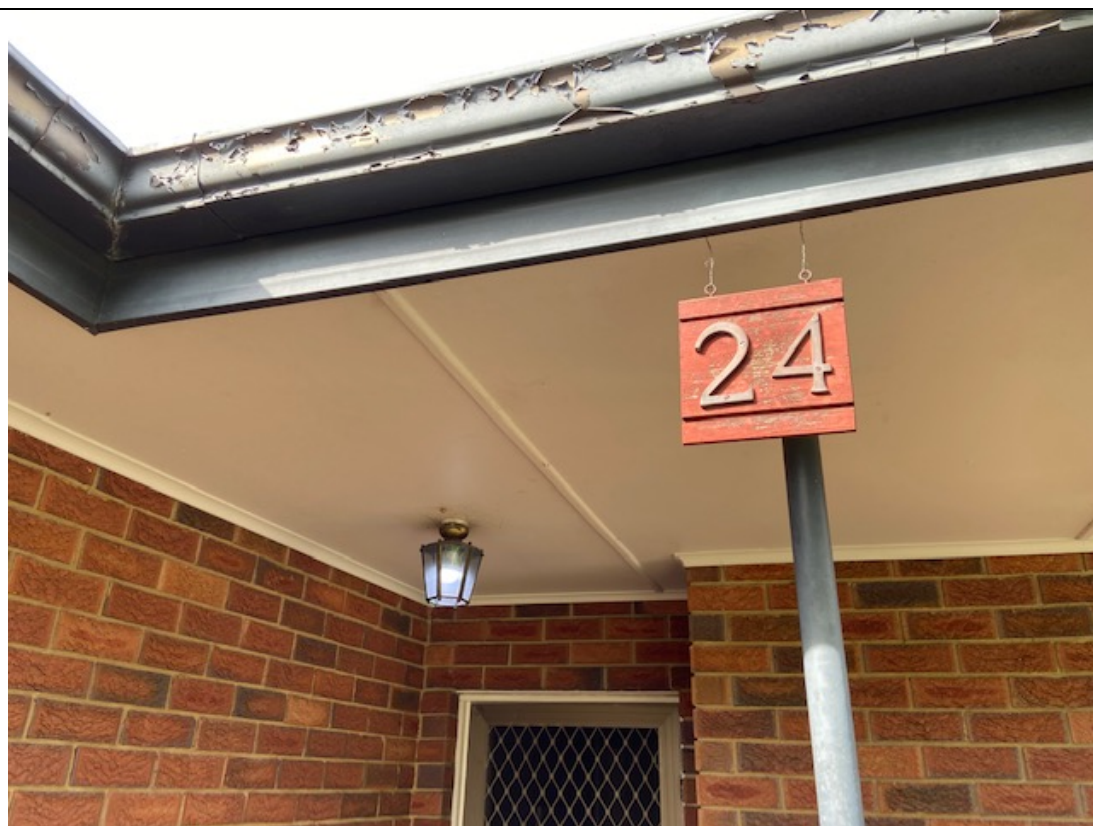
Photo 8 – Representative Construction Materials Used to Existing Site Buildings; Suspected Asbestos Containing Building Materials (as Fibro Cement Sheeting) Present to Areas of Built Structures at the Site
