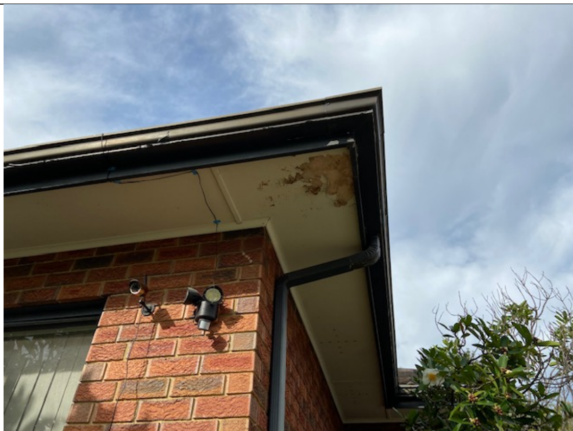
Photo 9 – Representative Construction Materials Used to Existing Site Buildings; Suspected Lead-Containing Containing Building Materials (as Paint System) Present to Areas of Built Structures at the Site
