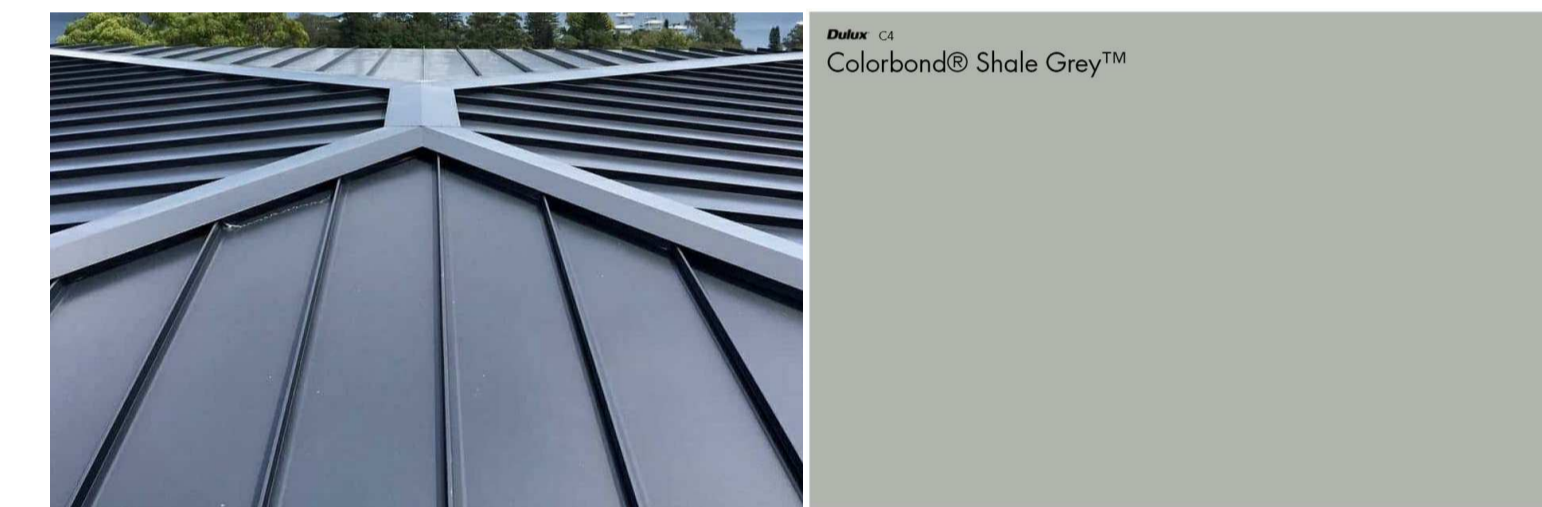
RF.01: STANDING SEAM ROOFING - COLOUR IN DULUX COLORBOND "SHALE GREY" C4 OR SIMILAR
