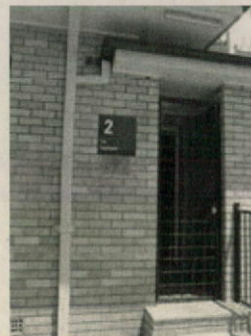
Photograph: View of existing signage "The Chambers" at entrance of the subject building.
