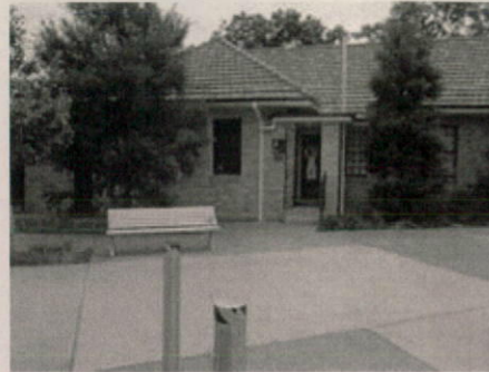
Photograph: View of existing East elevation
