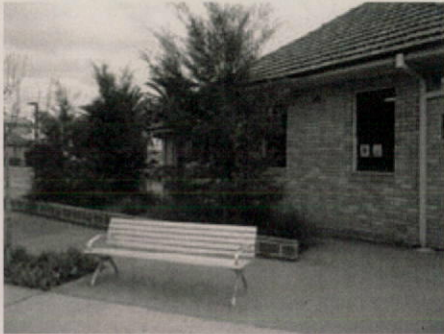
Photograph: View of existing windows on East elevation
