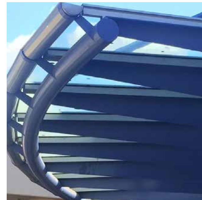
PAINTED METAL FRAME AWNING WITH GLAZING OVER
