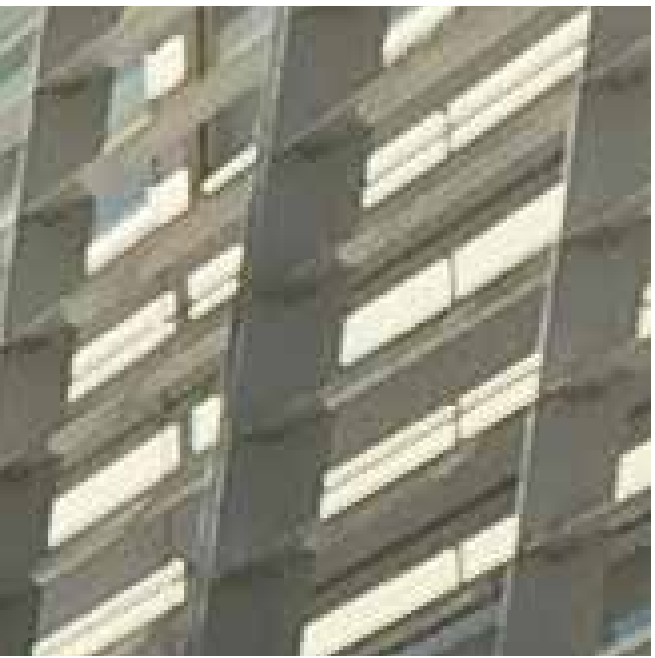
METAL LOUVRES IN HORIZONTAL ORIENTATION, FIXED TO METAL COLUMNS
