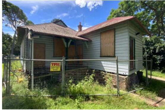
Figure 5: View of the rear elevation of the dwelling.
