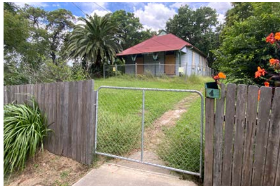
Figure 23: View of the front of the property facing south.
