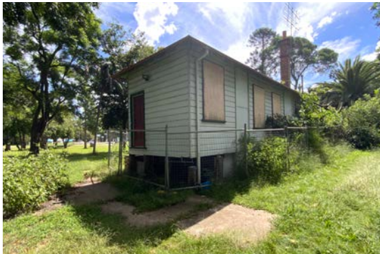
Figure 6: View of the eastern rear elevation of the dwelling.
