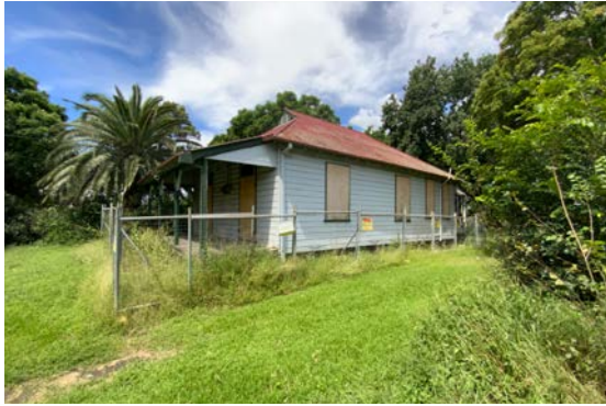
Figure 4: View of the western elevation of the dwelling.
