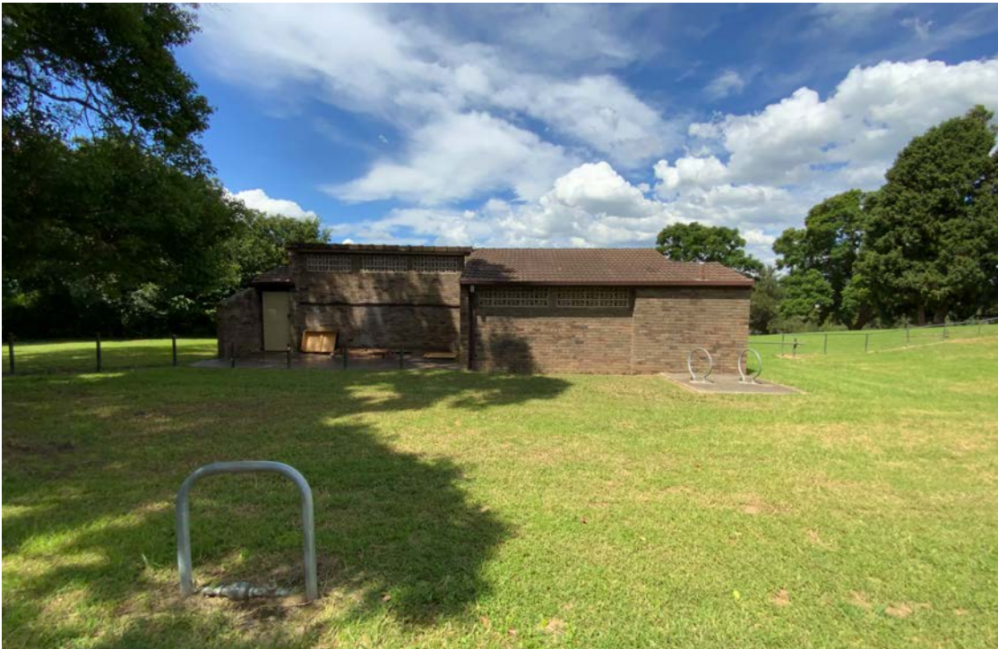
Figure 11: View of the amenities block situated on the eastern side of River Road.
