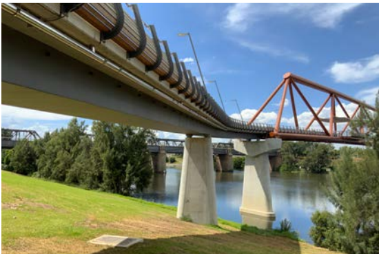
Figure 16: View of the former ferry crossing and the pedestrian bridge.
