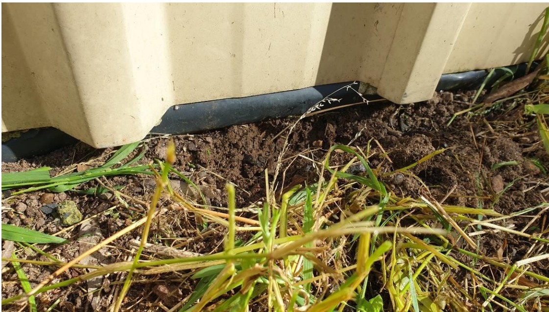
Figure 3: Image showing the plastic membrane under the slab
