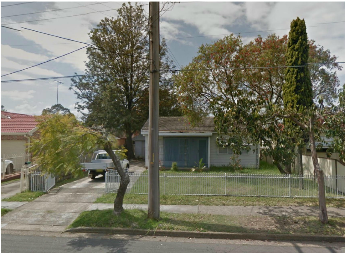
Photograph 1: Shows the subject site as viewed from Sydney St looking eastwards
