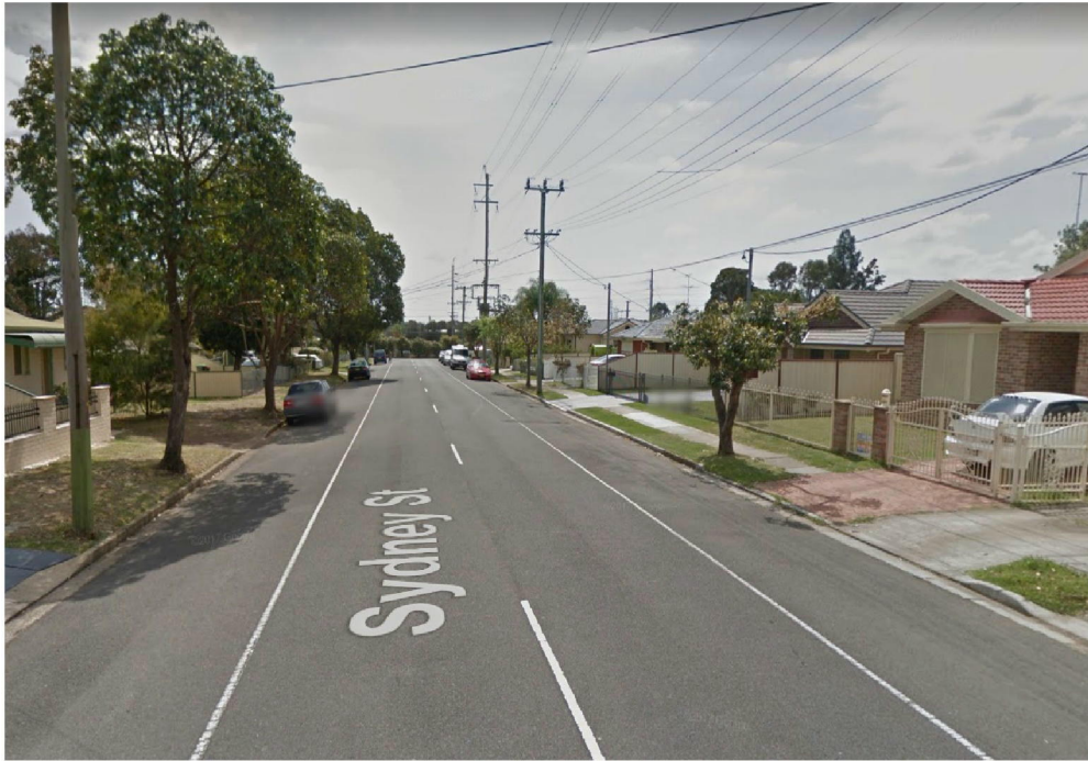
Photograph 2: Shows the existing streetscape along Sydney St looking northwards
