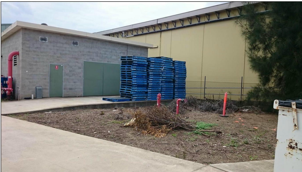
f) Proposed location for the new storage tanks.
