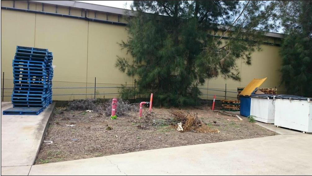
g) Proposed location for the new storage tanks.
