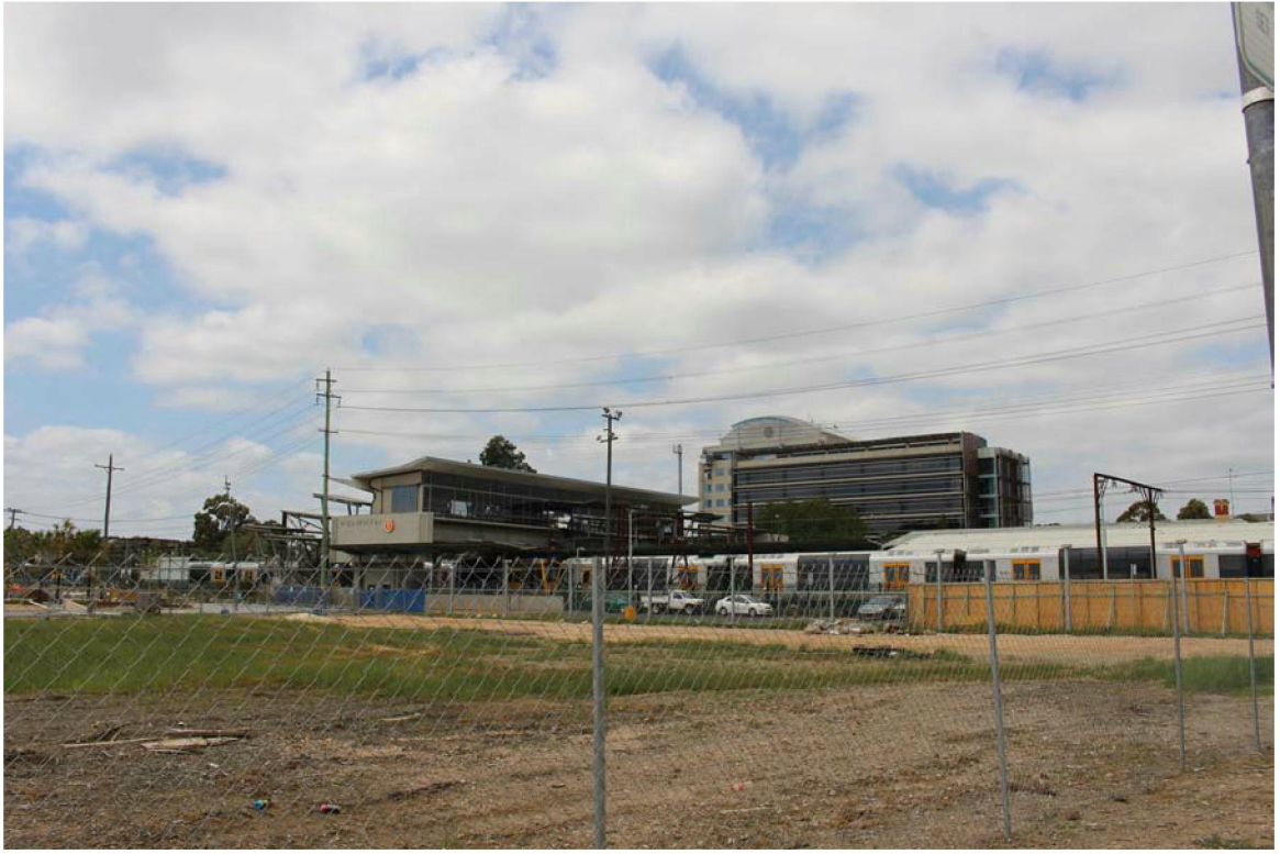
VIEW FROM DUNSHEA STREET TOWARDS PENRITH STATION
