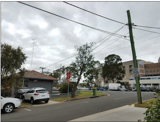
PHOTO 5 - HOPE STREET FRONTAGE
