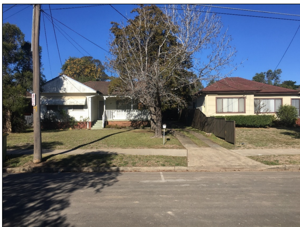
Figure 3b: Photograph of 18-20 Hope Street
