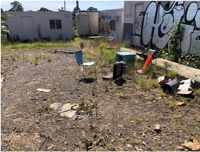
Photo 1: Work compound area with crushed rock hardstand surface
