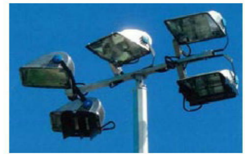
TYPICAL SPORTS LIGHTING LUMINAIRE ARRANGEMENT. INDICATIVE ONLY. FINAL LUMINAIRE TYPES AND QUANTITIES PER POLE TO BE CONFIRMED
