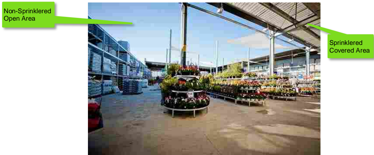
Figure 5 Example of the shade sails and open area of the garden centre with sprinkler omission.
