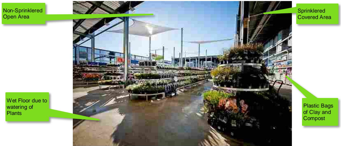
Figure 4 Example of the shade sails and open area of the garden centre with sprinkler omission.
