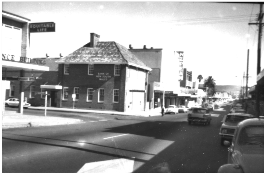
Figure 14: Photograph of the Bank of NSW, ca. 1970s. Source: Arthur Street, 'Bank of New South Wales, Corner High and Castlereagh Streets, Penrith,' ca. 1970s, Penrith City Library, https://penrithcity.spydus.com/cgi-bin/spydus.exe/ENQ/WPAC/ARCENQ?SETLVL=&RNI=325576 .
