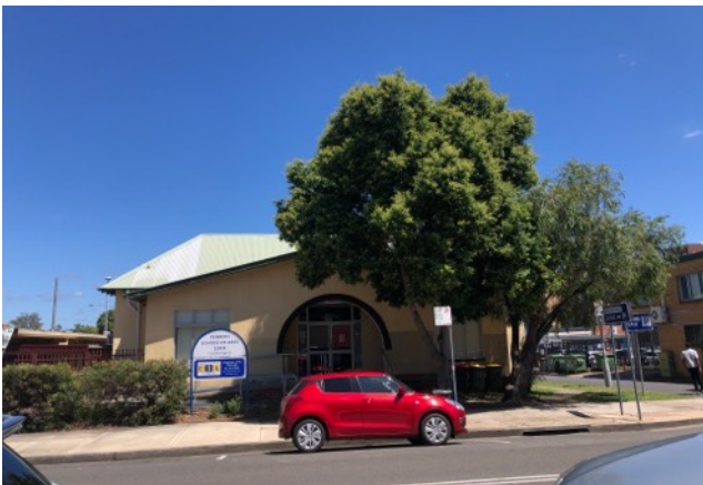
Image 16: Photograph taken on the eastern side of Castlereagh Street, facing west towards the heritage listed former Penrith School of Arts.
