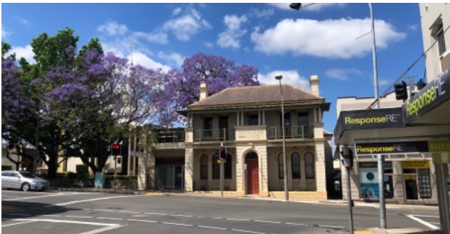
Image 5: Photograph taken on the western side of Lawson Street, facing south towards Cram Place and the subject site (visible behind Cram Place and to the right of the image).
