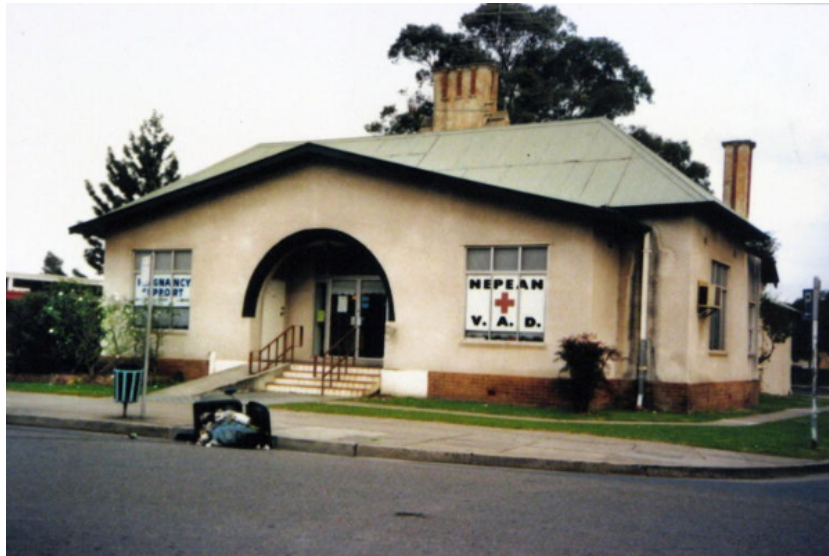
Figure 16: Photograph of the Penrith School of Arts in the 1970s, after extensive changes were made to the front façade. Source: Gerald O'Farrell, 'School of Arts, Castlereagh Street, Penrith,' ca. 1970s, Penrith City Library, https://penrithcity.spydus.com/cgi-bin/spydus.exe/ENQ/WPAC/ARCENQ?SETLVL=&RNI=316054 .
