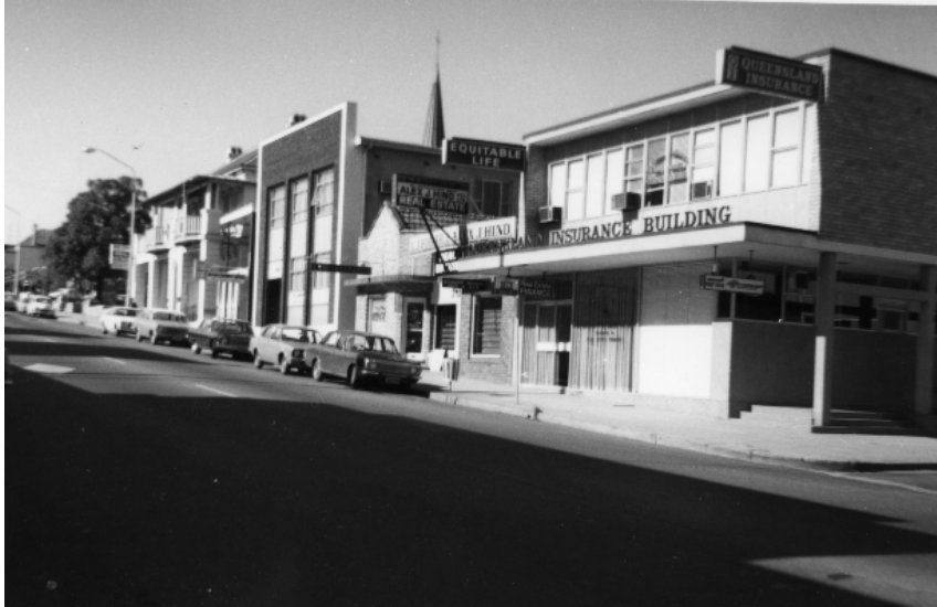
Figure 10: Photograph of High Street from the intersection with Castlereagh Street, ca. 1970s. The buildings at 342-346 High Street have been demolished and replaced, while 348 High Street remains the same. Source: Arthur Street, Penrith City Library, 'High Street, corner Castlereagh Street, Penrith,' ca. 1970s, https://penrithcity.spydus.com/cgi-bin/spydus.exe/ENQ/WPAC/ARCENQ?SETLVL=&RNI=327361 .
